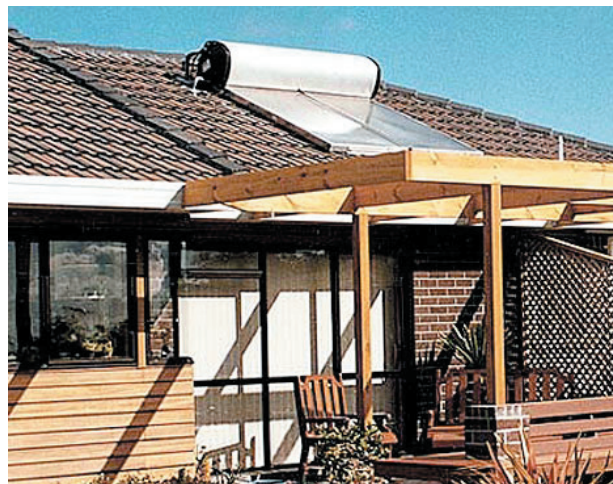
Use of a solar hot water panel on North-facing roof
