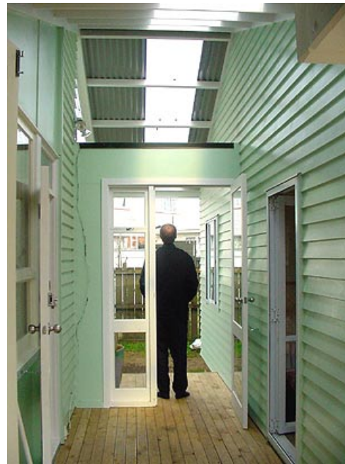
View through new rear entry linking existing house with connected wing
