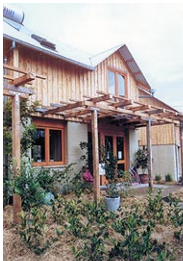
Earthsong eco houses showing use of energy efficient principles such as thermal mass in the lower storey, solar water heating, permeable pergolas for summer coverage by seasonal climbing plants, use of natural materials, opening skylight for light and ventilation.
