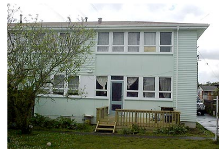
Rear yard / west elevation
