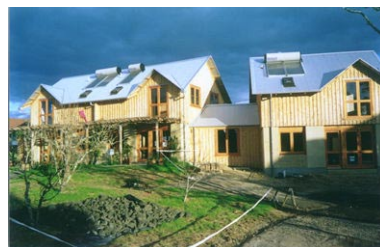
Earthsong eco houses showing use of energy efficient principles such as thermal mass in the lower storey, solar water heating, permeable pergolas for summer coverage by seasonal climbing plants, use of natural materials, opening skylight for light and ventilation.
