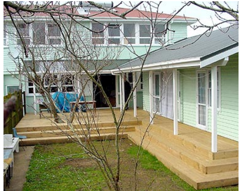
View of new north-west facing verandah linking existing house with connected wing
